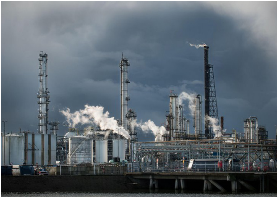
The Shell Oil refinery in Pernis, the Netherlands
